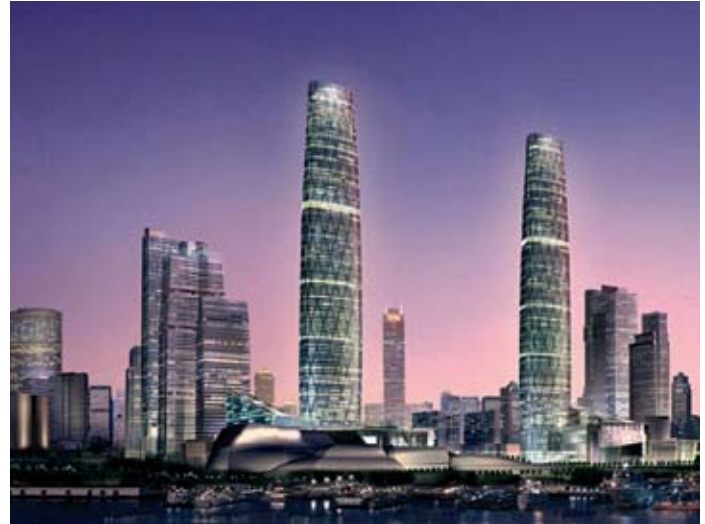
Guangzhou Twin Towers
